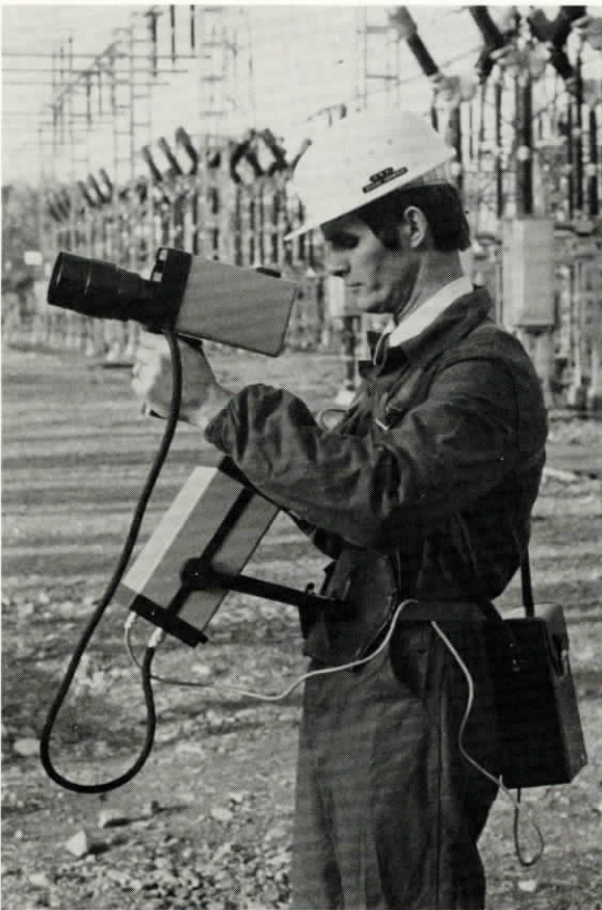
A remote infrared sensor used to obtain a thermal image of stand-off-insulators on a power transmission line. Points of potential failure appear as hot spots on the thermogram.
