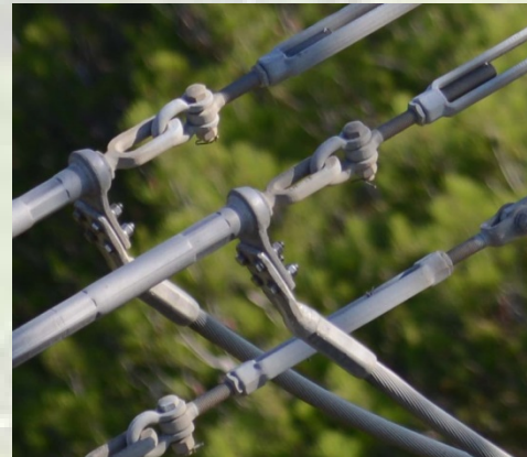
Picture to the right shows cotter pins in place and hardware secure!>>
