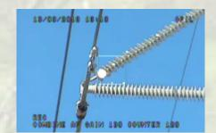
Contaminated insulators and bushings can create havoc with the delivery of our electricity! Dirty or damaged insulators are susceptible to Electrical Corona and Arcing causing flashover & downed lines.
