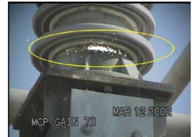
The two pictures to the right show severe Corona on a **NCI Polymer Insulator**. The left picture vividly shows the Corona discharge with medium gain of 180. In the right picture the gain has been reduced to **pinpoint the exact location of the problem!** Observe the high Corona photon count. This insulator needs to be replaced and the replacement unit needs a corona ring! The camera gain setting goes from 0 to 250.
