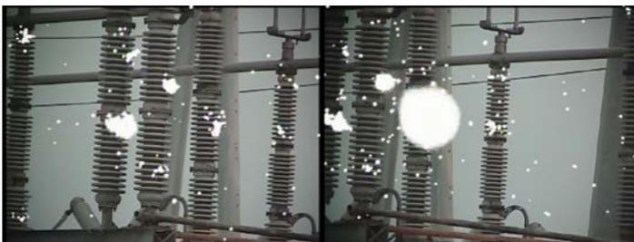
The pictures **to the left** shows Corona on buss support insulators with a **high level of contamination**. To prevent a flashover event, cleaning or washing of insulators is needed! Part of the corona seen is due to **dry-band arcing**. The detection of corona and its **precise location** is very important information for the utility professionals and cleaning crews.
